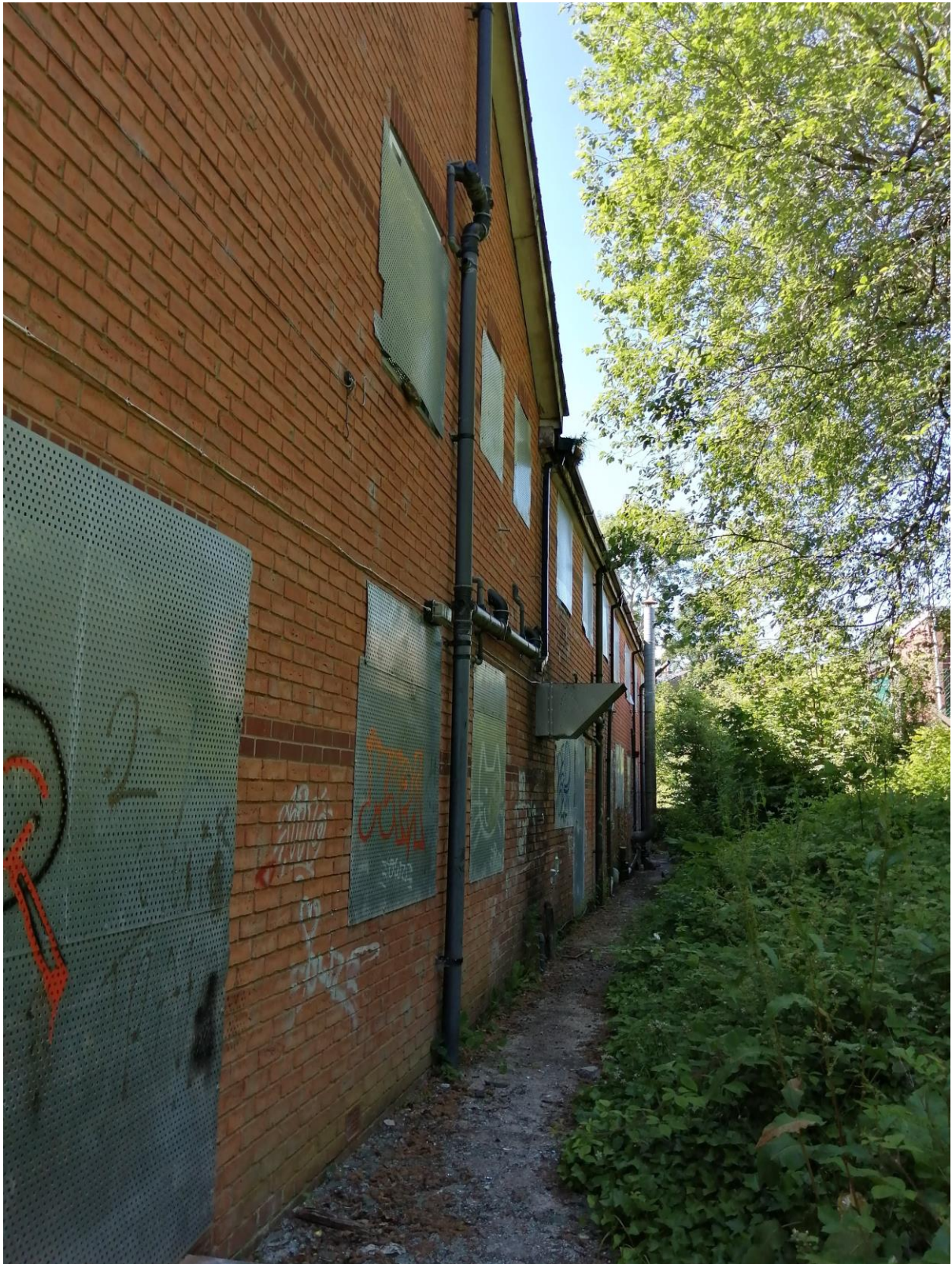
Photo 4: The eastern elevation of the existing building
