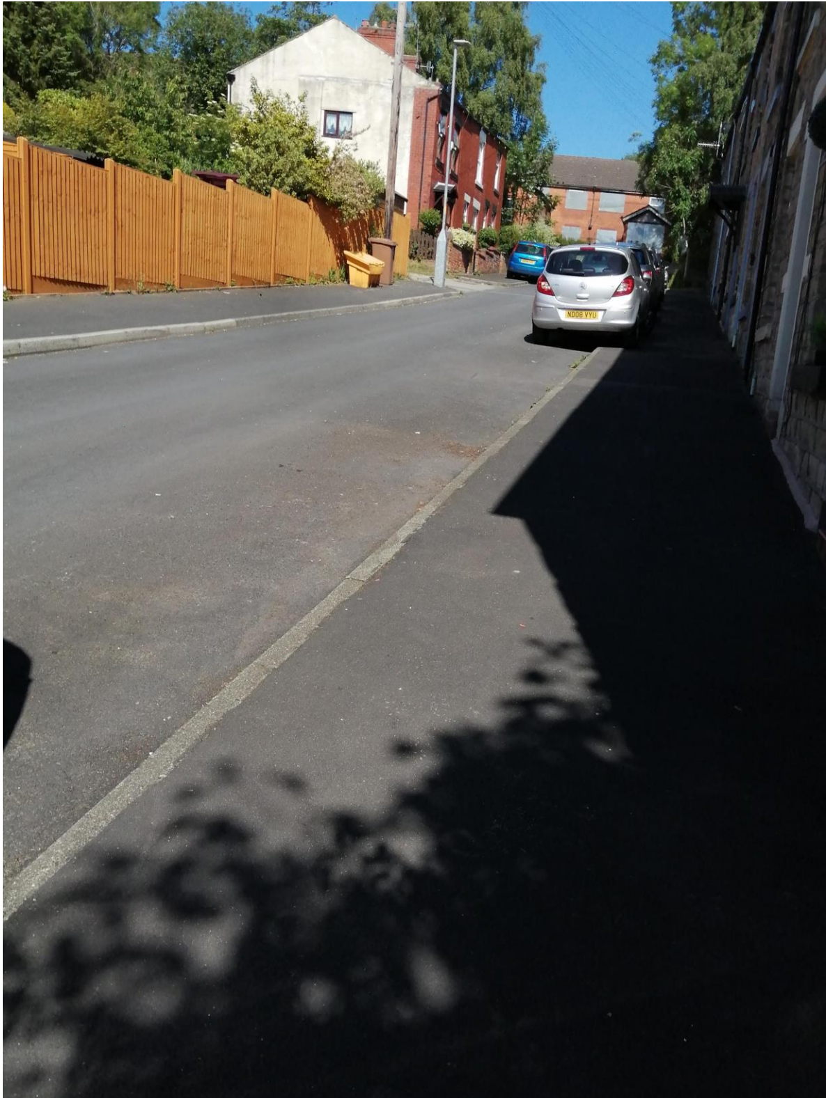
Photo 1: View of the site from Duke Street
